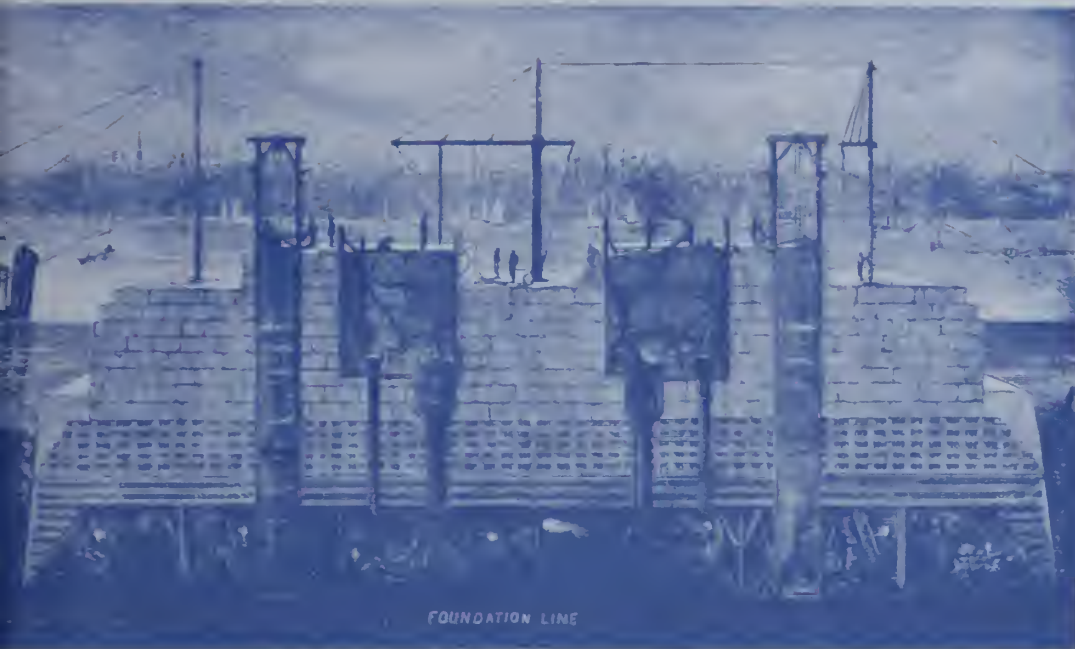
Sectional view shows method of excavating under caisson while the courses of stone for the pier are built up, their weight gradually pressing the caisson down to a depth of 45 feet below mean high water on the Brooklyn side.
